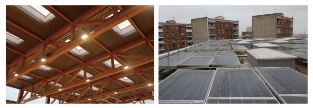
Figure 62-63. Motorized skylight and rooftop photovoltaic panels.
