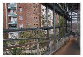
The building is mostly wrapped with a highly durable polycarbonate façade, which creates pockets of air for building insulation and filters the natural light due to its translucent nature. The south-facing façade has an additional layer of curtain wall made up of hydroponic plants. It controls sunlight depending on the season and is watered by the building's rainwater reuse system.
